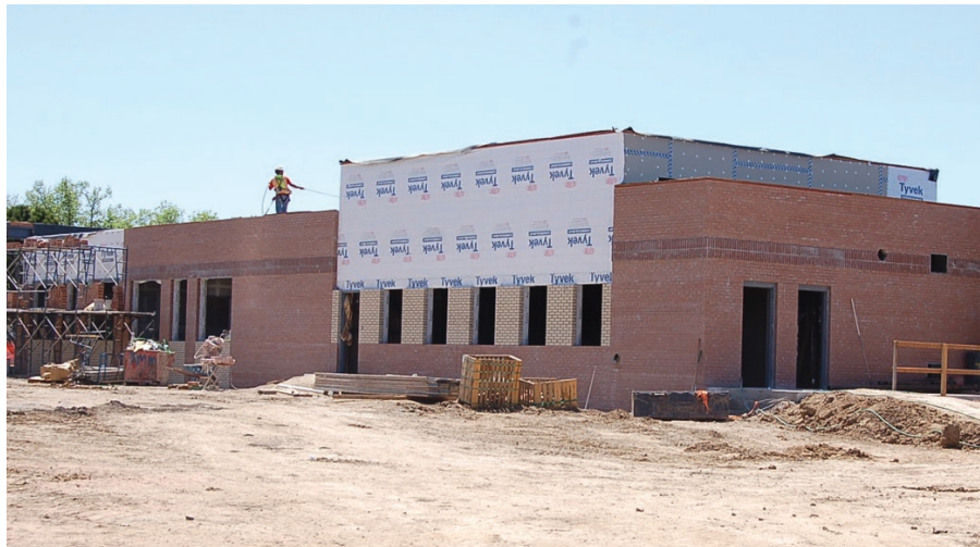
Construction progresses on additions to Elkhart Elementary School.
