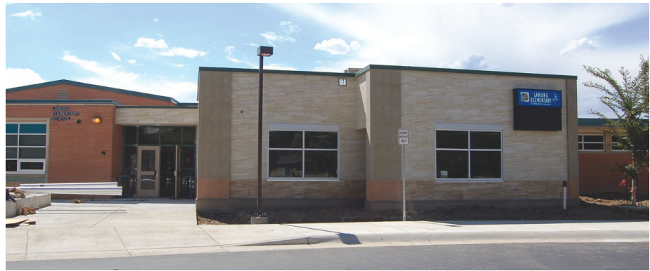
Lansing Elementary features a new front entrance addition.
